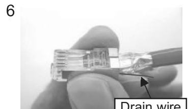
6 Insert the cable into the modular plug so that the folded part of the shield enters into the plug housing. The drain wire should be located on the tab side of the jack.
