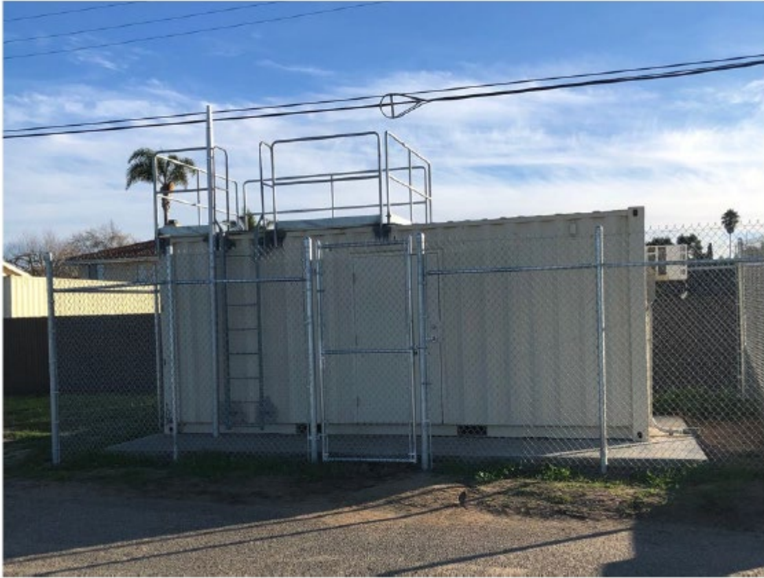
Figure 3: Station Building from the Front
