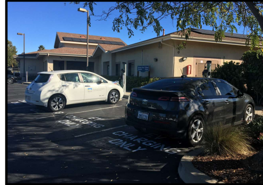
Infrastructure (Santa Ynez Chumash)
