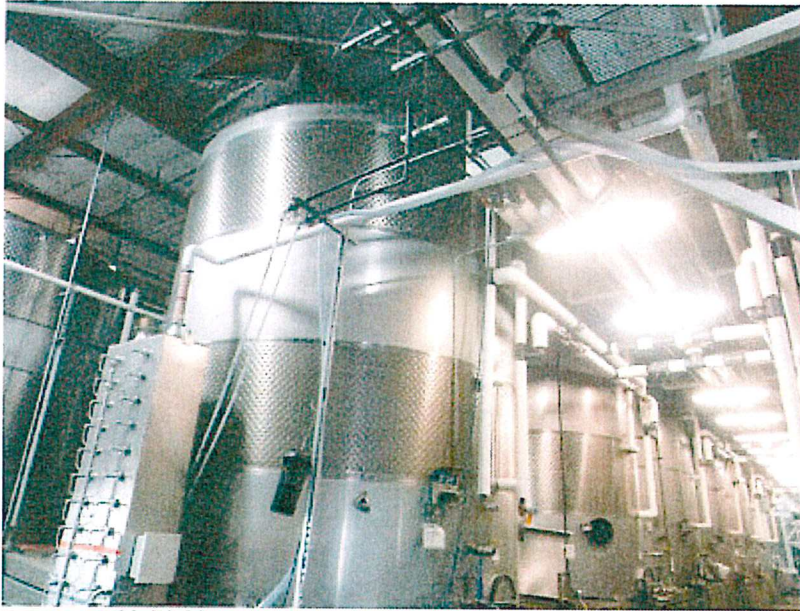
NoMoVo control system with NoMoVo piping manifold
