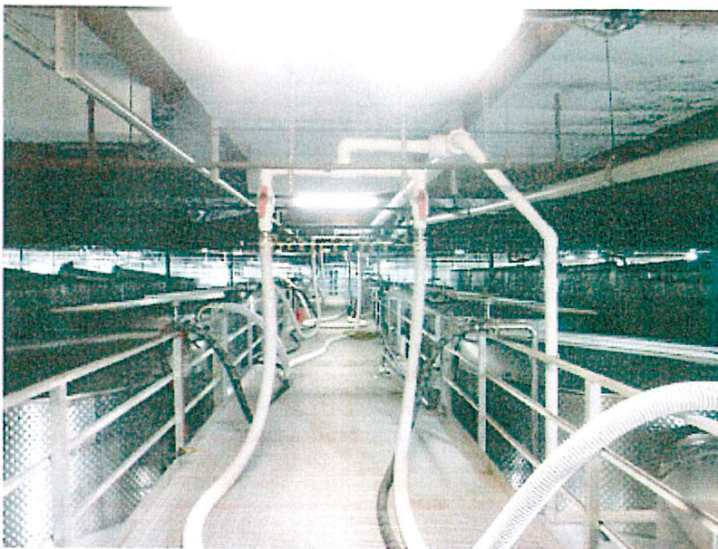
Closed top fermentation tanks with NoMoVo piping manifold
