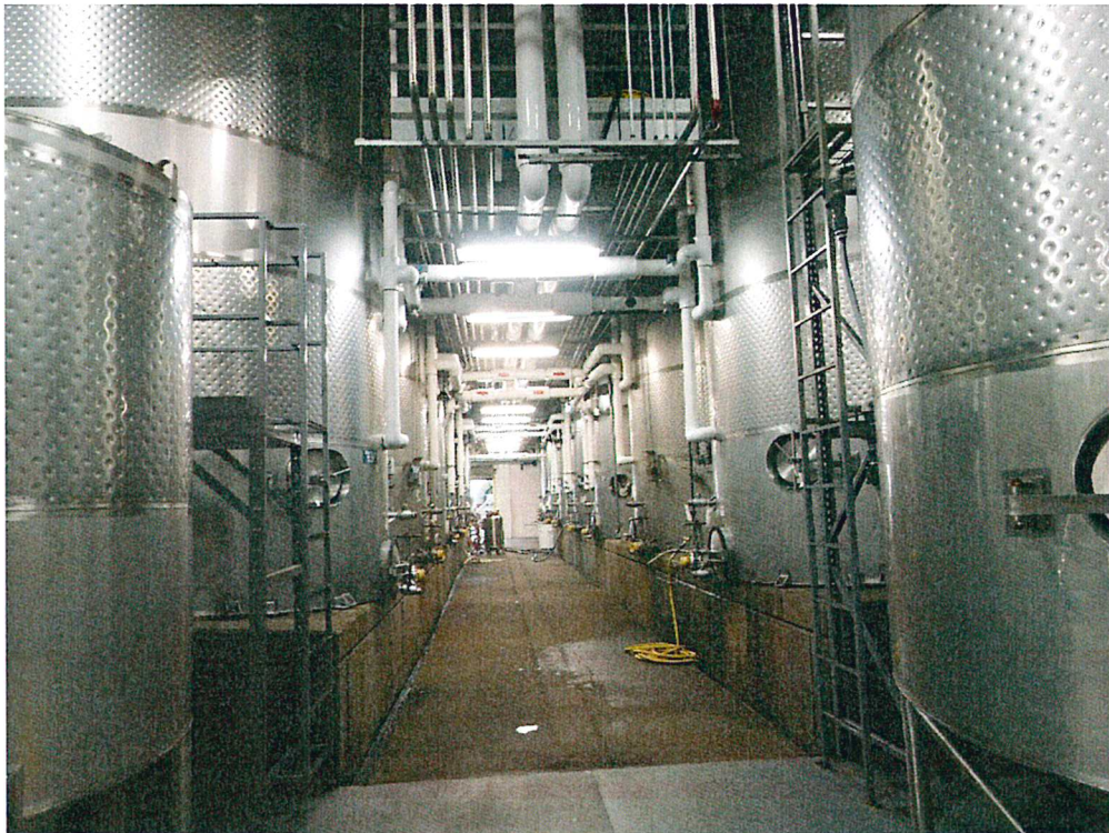
CCWS Series 400 tanks and EcoPAS piping manifold
