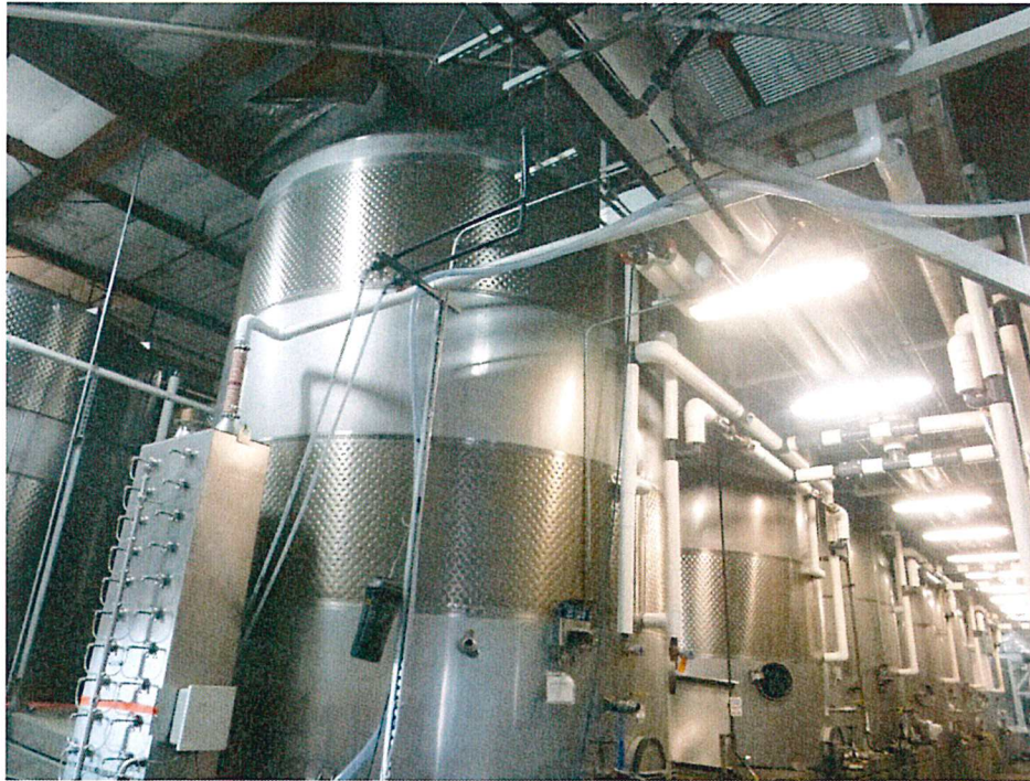
NoMoVo control system with NoMoVo piping manifold
