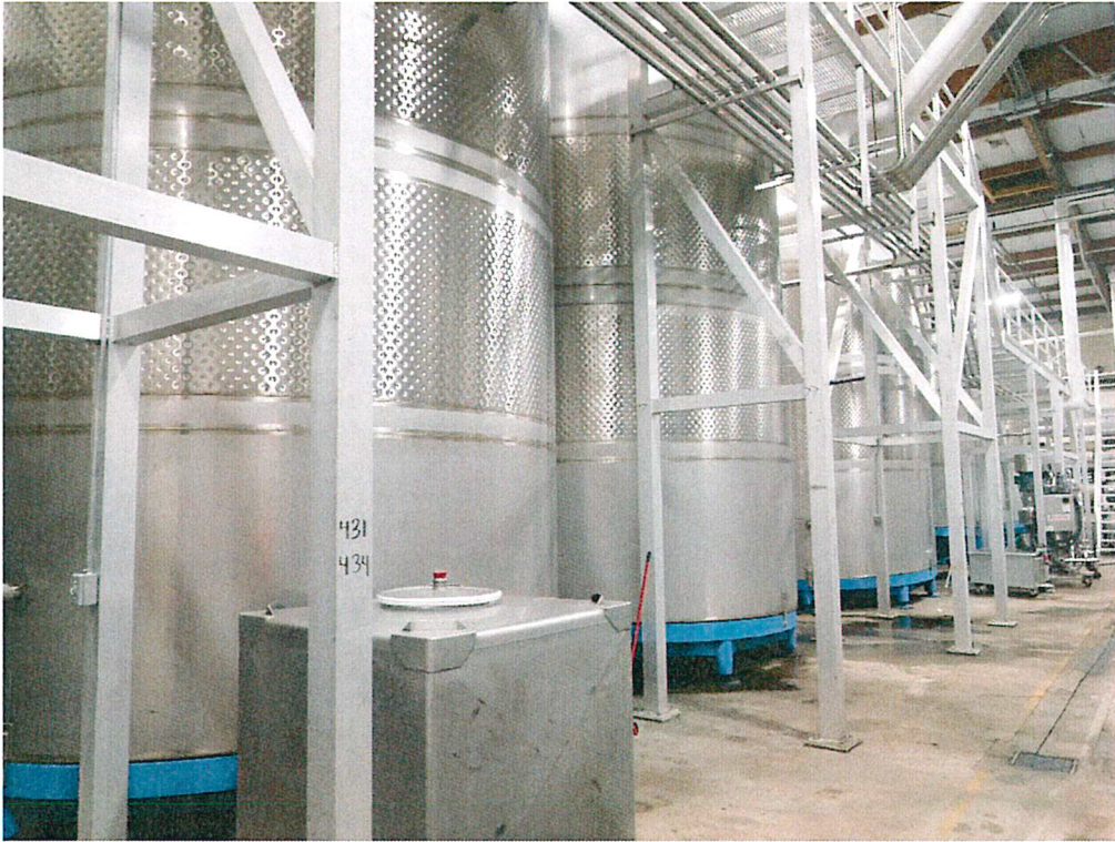
CCWS Series 400 tanks and EcoPAS piping manifold
